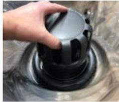
Pull Up to Remove Floater Assembly
